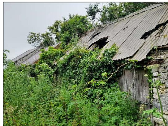
Plate 4-8 External view of the sheds, showing missing sections of roof and damage
