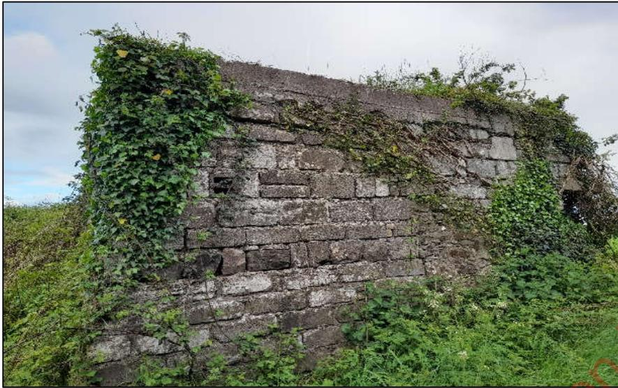
Plate 4-2 Derelict Stone building showing ivy cover and gaps in the stonework with *Low* potential.
