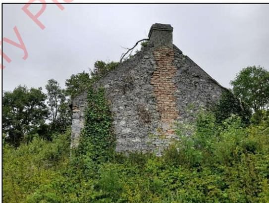
Plate 4-7 Stone and block house, missing roof sections.
